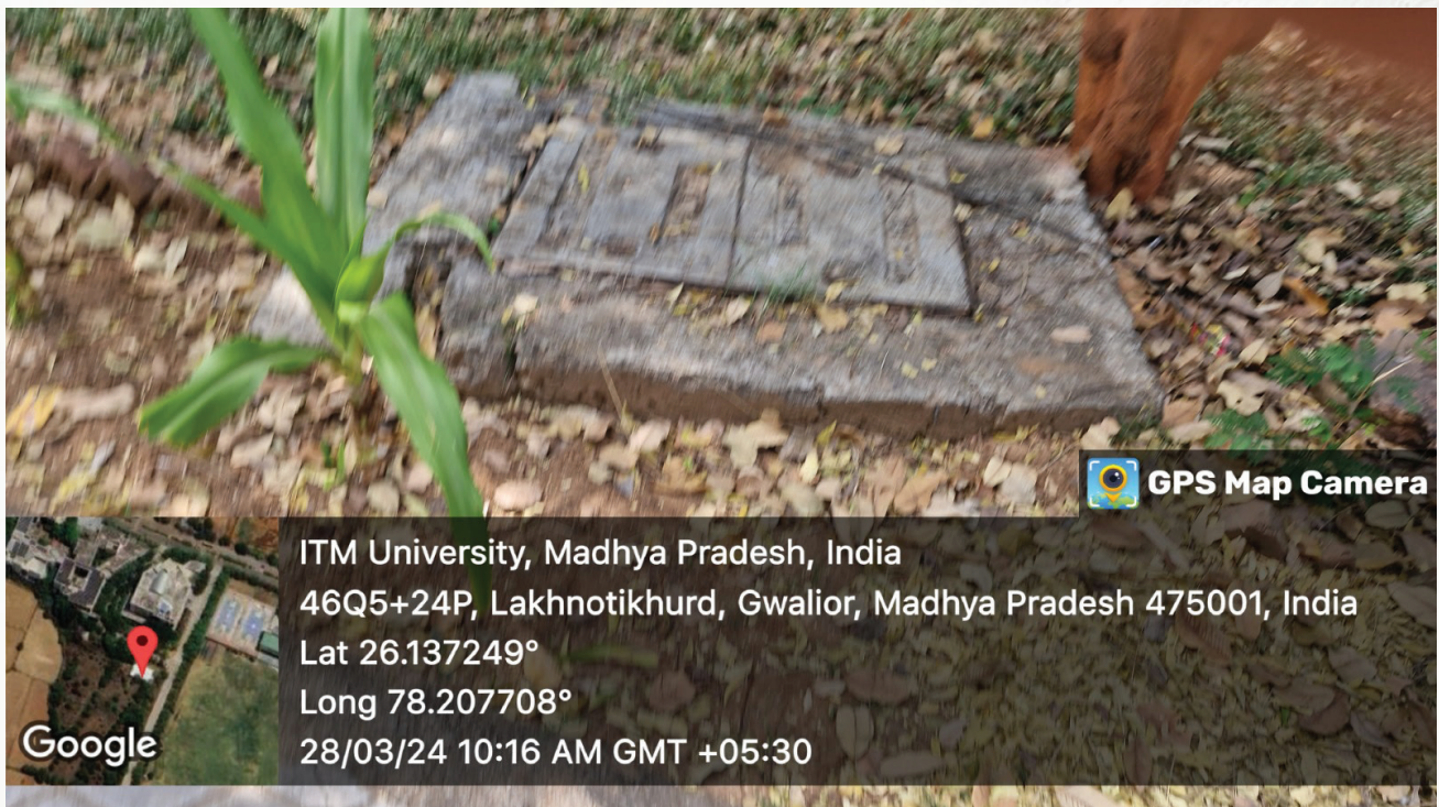
Septic tanks at various places in campus
